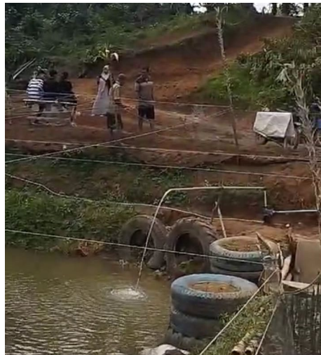
Figure 3. Pump on after all components have been assembled.
