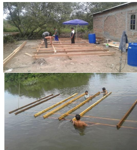
Figure 1. Installation of floating net frames
