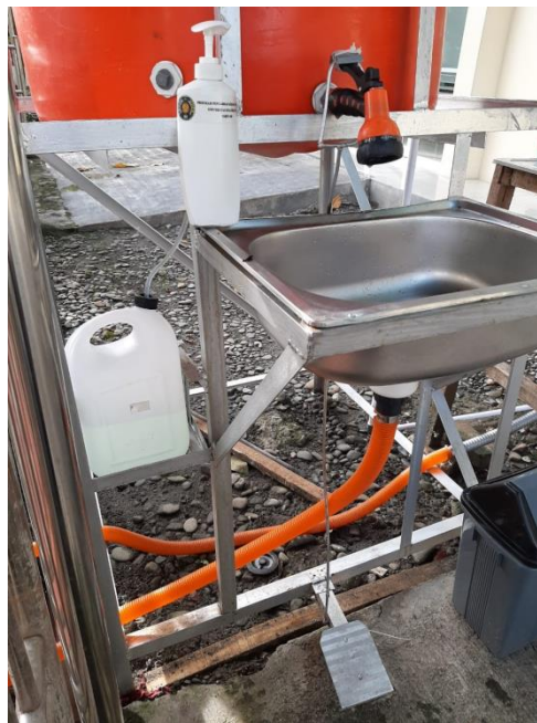
Figure 5. Foot pedal position in the hand wash basin
