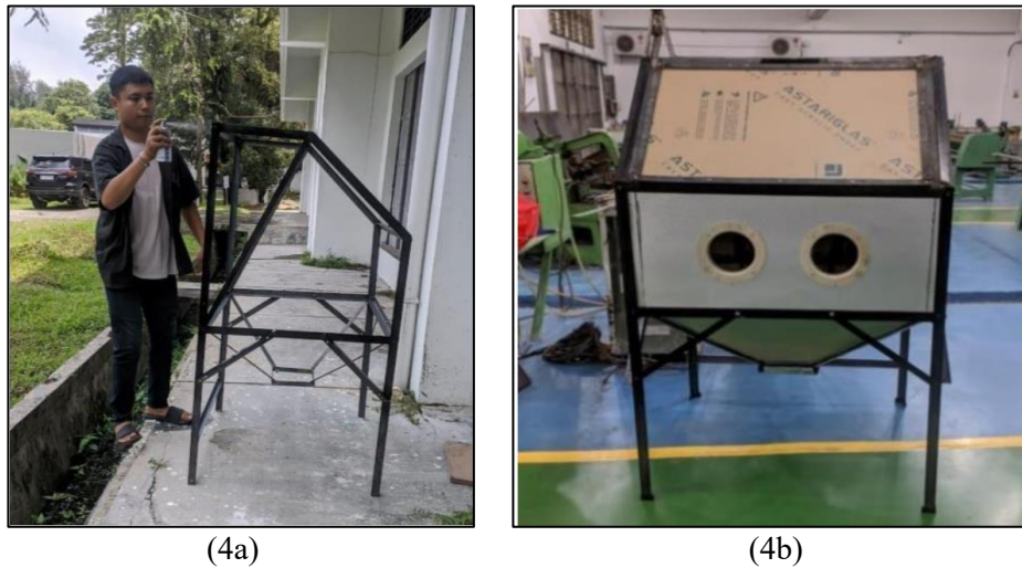
Figure 4 (4a) Frame Coating ; (4b) Installation of Cover Plate and Acrylic Pane
