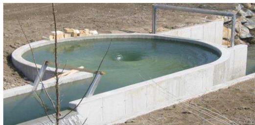
Gambar 2.5 Turbin vortex Zotloterer
