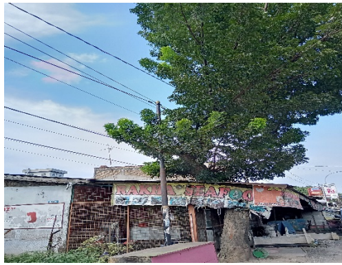
Figure 6. Mahogany trees ( Swietenia mahagoni ) pose a threat to the home and cables
