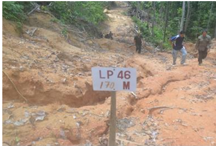
Figure 1. Soil erosion on the slope of a skid trail due to heavy rainfall. (JPSM, 2014).
