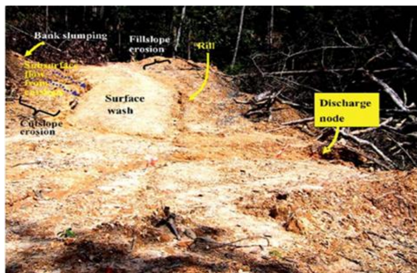
Figure 2. The rill and gully erosion on a forest road in Malaysia. (Sidle et al., 2006).
