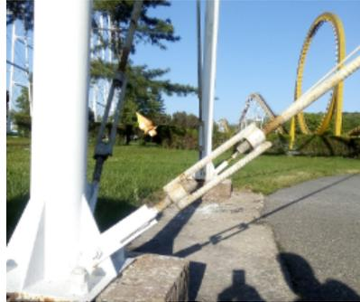
**Figure 8** The Brace With Turnbuckle
