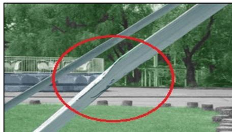
**Figure 6** Deformed Bar With Buckling When it Compresses
