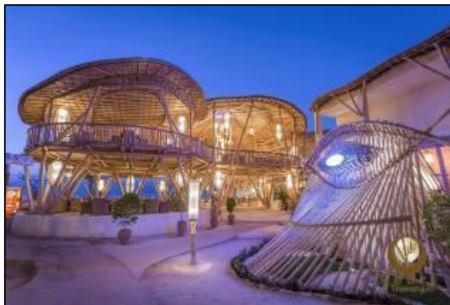
Figure 1. Pearl Beach Lounge', Gili Trawangan, Lombok
