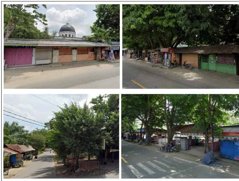
Figure 3. Existing Building Condition Source: Google Earth [16]
