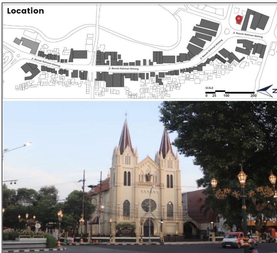
Figure 2 Catholic Church of the Holy Heart at the End of the Road Kayutangan
