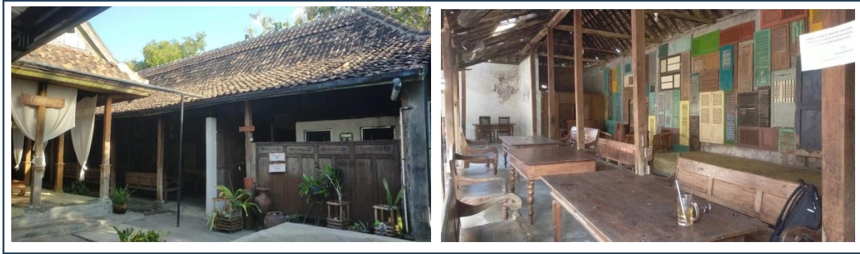
Figure 14 Joglo and current bathroom area Source: Personal Documentation
