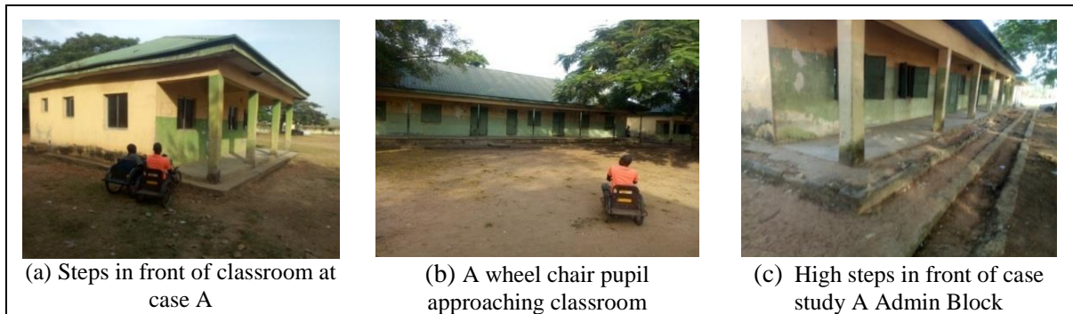
Figure 4. Classroom with steps
