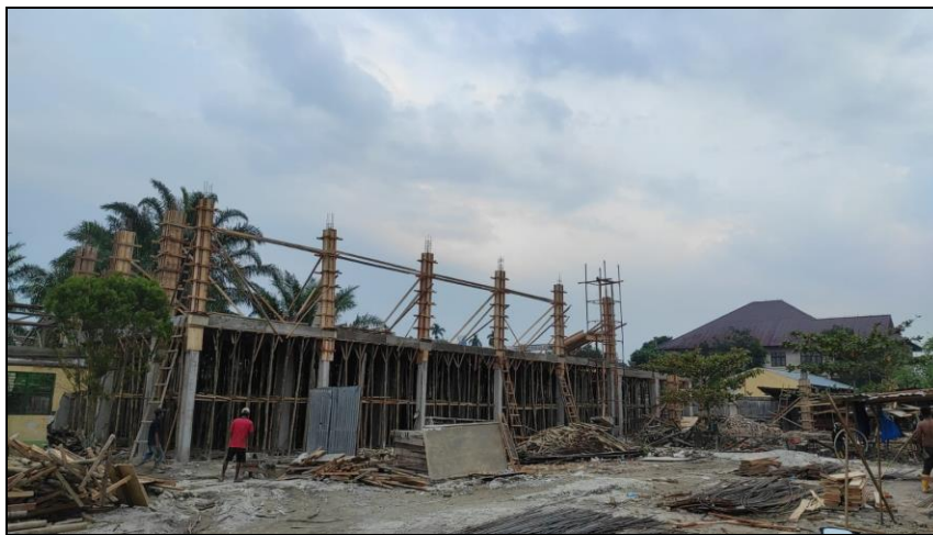
Figure 1 New classroom Construction project at SMPN 31 Medan (Source: primary data, 2023)
