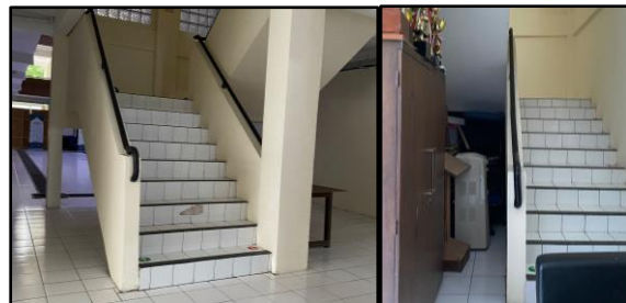
Figure 6 (a) Main Stairs; (b) Side Stairs Source: (Direct Observation, 2024)
