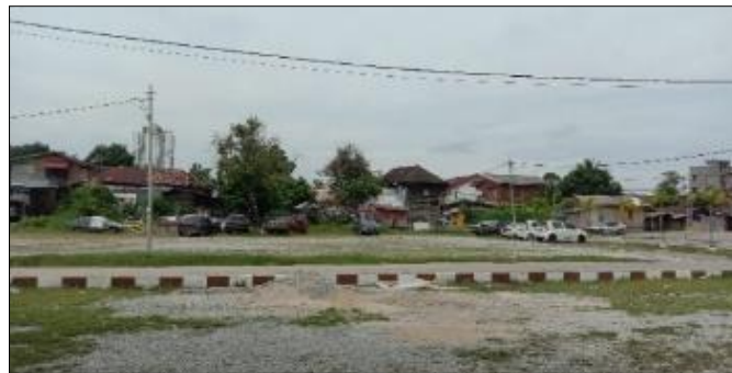
Figure 5 Atas Paloh Village after demolition works (Fieldwork, 2019)
