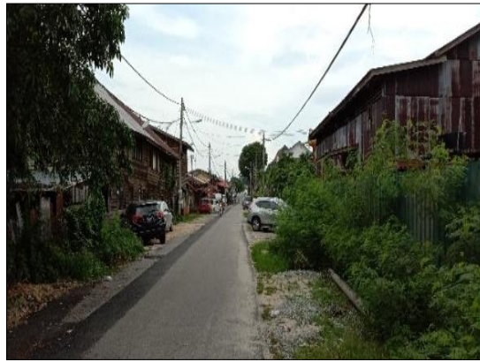
Figure 8 The picture shows a settlement in Pengkalan Pasir Village before the demolition work
