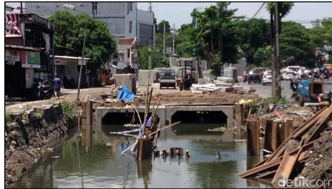
Figure 2. The box culvert development project in Jemur Ngawinan street, Surabaya [3].
