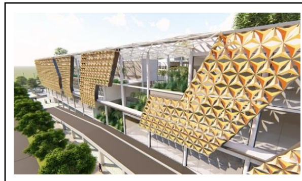
Figure 7. Metal secondary skin as a buffer
