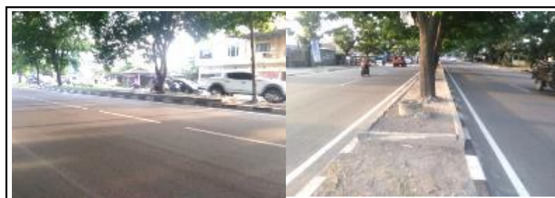
Figure 3 Types of Median Road Applied on Jalan Asrama, Medan
