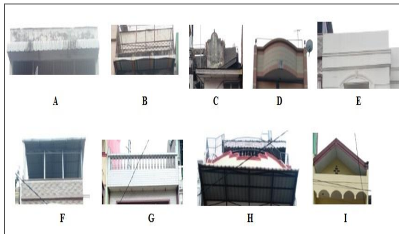
Figure 5 Type of Roof
