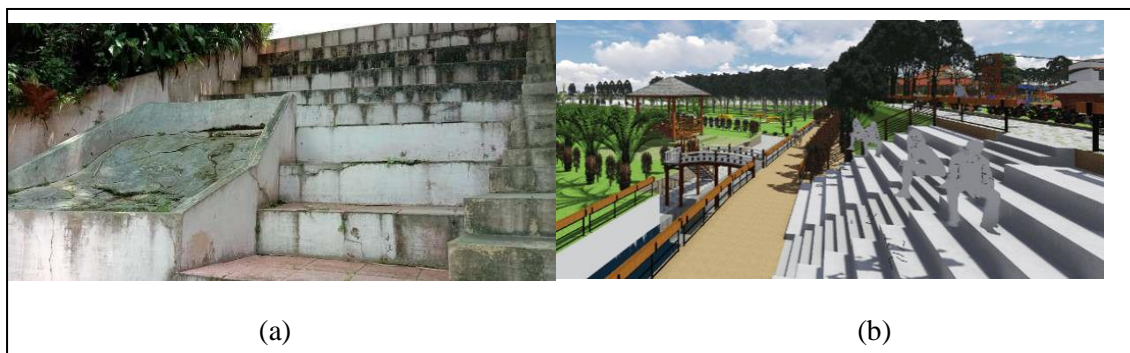
Figure 5 (a) Stairs before being revitalized, (b) Stairs after being revitalized
