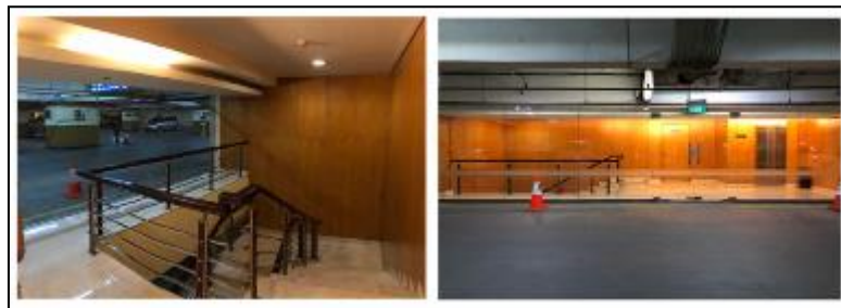
Figure 11 Elevator and Stairwells
