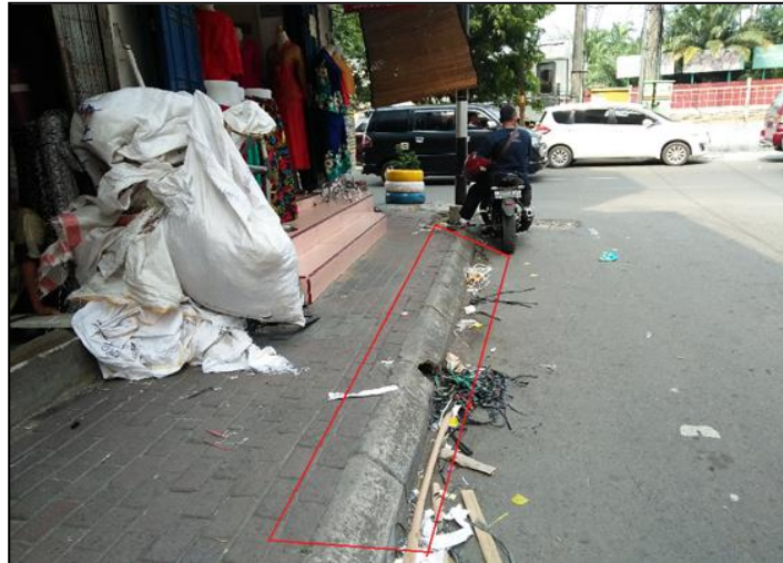
Figure 6. Elements of Edge at Perniagaan street – Roadblock and Drainage
