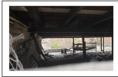
Figure 3 Substructure for livestock
