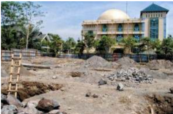
Figure 1. Excavation Stage (Source: Kemendikbud, 2014 [2])
