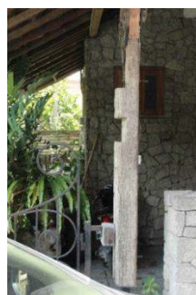
Figure 11. Stone Wall as Facade (Source: Author Archive)
