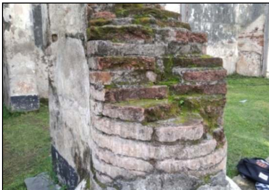
Figure 4. A material of the walls of the fortress of Van Den Bosch uses red brick
