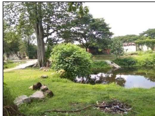
Figure 2. A trench that does not already function again
