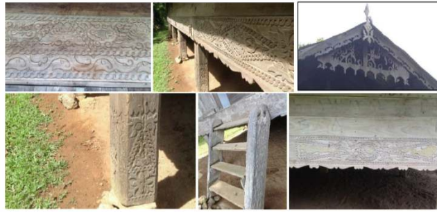
Figure 6. Decorative elements on traditional Gayo Lut house
