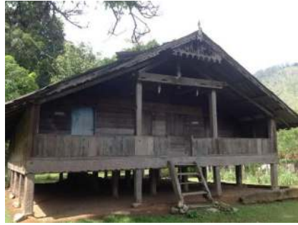
Figure 3. Traditional Gayo Lut house in kampöng Toweren in 2015
