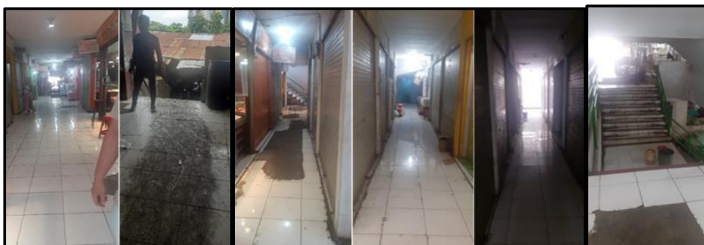
Figure 4 The condition of the first floor of the Sukaramai Medan Traditional Market
