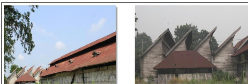
Figure 2 The facade of former PTPN II tobacco ripening warehouse
