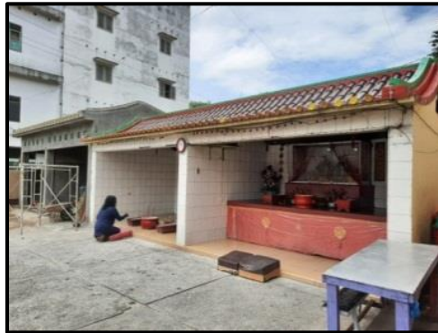
Figure 6 Side Building of Maha Dana Temple
