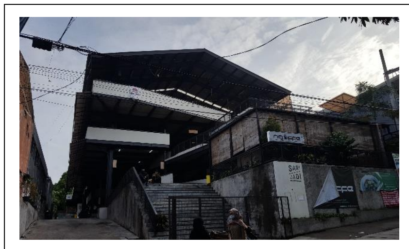
Figure 11 Facade of Sarijadi Contemporary Market
