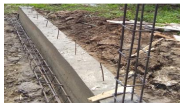
Figure 9. Foundation after being casted
