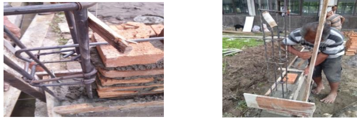
Figure 13. Angkur Installation Details
