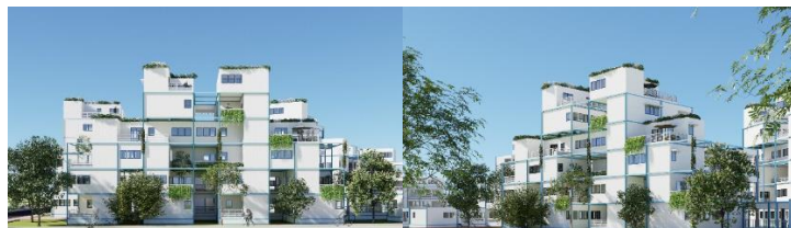
Picture 9. Building Exterior Source: Personal Data, 2023
