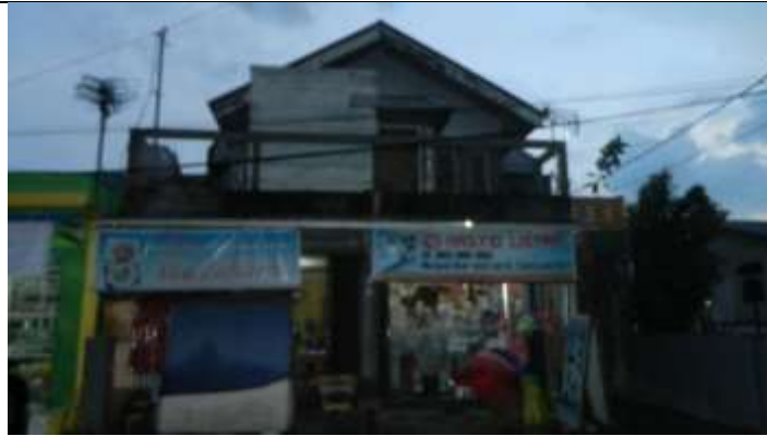
Figure 2. Photograph of the converted house (Typology A: complete conversion sample).
