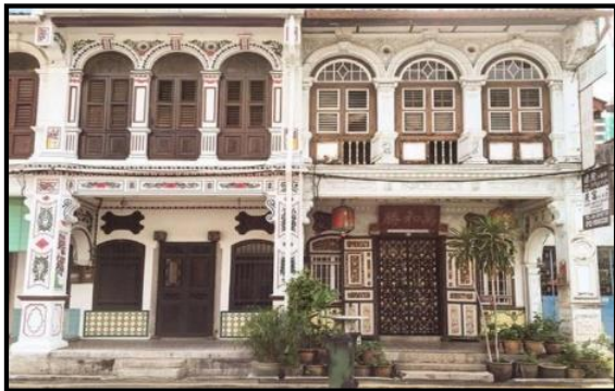
Figure 2. Chinese Shophouse Facade
