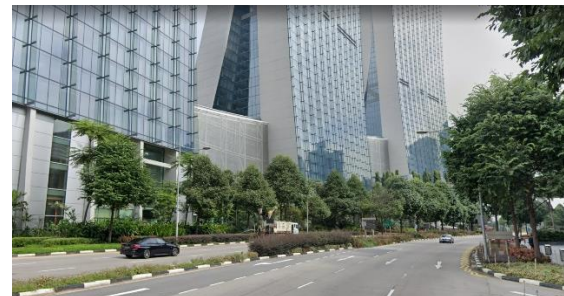
Figure 6. vegetation on the front of the building. (source: www.googlemaps.com )
