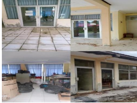
Figure 4.2 Condition of UPTD P2PMKS Nilam Suri
